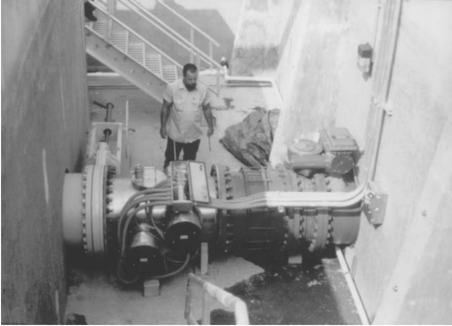
FIGURE 99 Disinfection of wastewater at Gwinnett County, Georgia. Total flow = 1580 \text{ m}^3/\text{h} , T_{10} = 74\% . Each of four reactors is equipped with 16 medium-pressure lamps.
