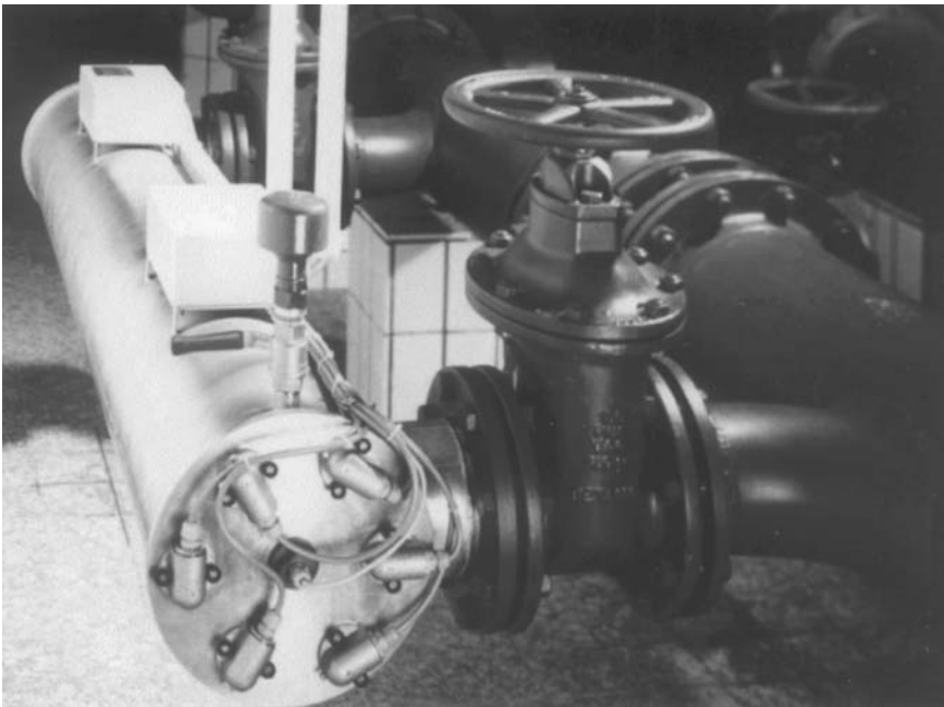
FIGURE 75 Six-lamp reactor at Gelsenwasser, Germany. Installation Wedeco.
